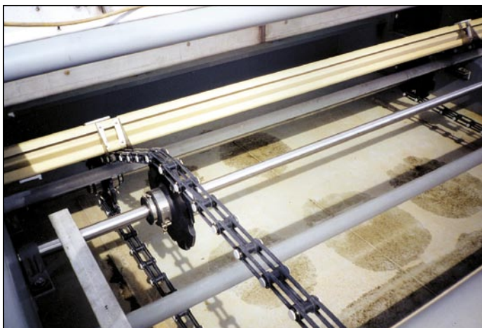
FIGURE 6. In many cases, the components for modern chain and flight collectors employ fiberglass as a material of construction
